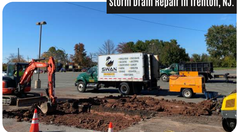
Storm Drain Repair in Trenton, NJ.
